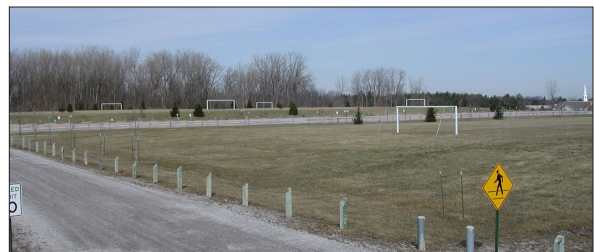
Saturday morning soccer games are played on the site of the former Linden Road Landfill. A restrictive covenant is recorded on the property deed to prohibit excavation or other soil disturbance activities below the cover.
